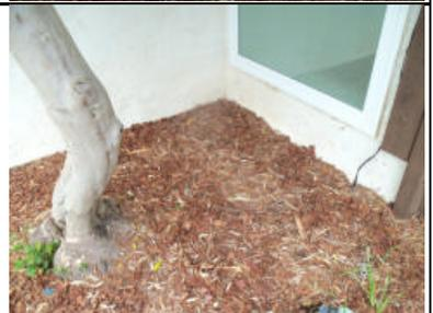
[CR] This picture shows how high the soil level is in relation to the floor level of the pool house. The soil level is too high all the way around and needs to be lowered and the area around this building re-graded. The soil level needs to be a minimum of 6 inches below the slab level. This will be a substantial task.
