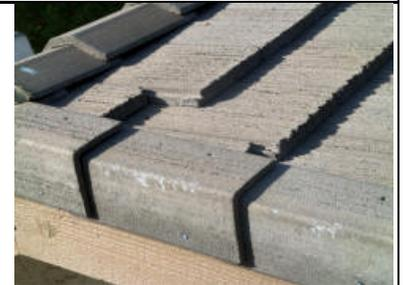
This picture is over the master bath. The tile was not secure along the edge of the wall and moved.
